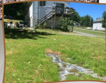
Failing septic systems
